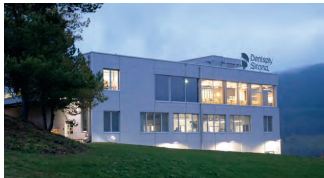
Our facility in Ballaigues, Switzerland uses 572 photovoltaic panels (930 m 2 ) implemented on the roof delivering 151.6 kWp.
